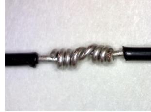
Figure 19-17. Completed Wrap for Western Union/Lineman Splice
